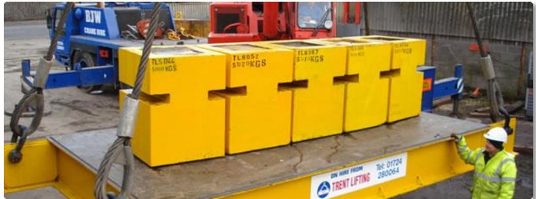
Knowing the load weight is important to preventing accidents with the lift.
