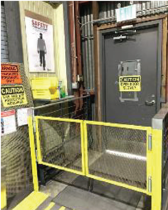
PPE Station example (Picture Courtesy of McKinstry Co.)
