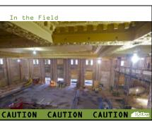
One of the largest safety issues during this phase of construction was the air quality. Without proper ventilation (shown here with fans in the windows, openings for cross ventilation, and a large filter bag in the lower right of this image) the 12 welders would be creating a lot of toxic air for themselves and other trades to breath.
