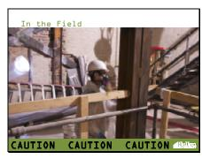
Low level lead based paint was one issue, shown here, it's being removed with a gel product so welders can reinforce these steel columns and not inhale the lead while welding
