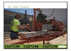
In this particular case, the project team decided to take their deconstruction, salvage, and reuse practices a step further by bringing a portable mill onto the jobsite to mill reclaimed lumber for immediate use including the creation of formwork for the rest of the project.
