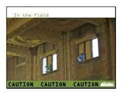
Ventilation combined with daylight by using a translucent material instead of the common plywood.
