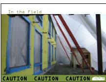
The image here is an example of a project that through IAQ Best Management Practices enabled the schedule to stay on track. By using temporary plastic in lieu of window systems that hadn't yet arrived, it was able to maintain the critical schedule and continue with the installation of interior drywall and insulation. The second layer of plastic was used for source separation of airborne particulates while soil grading was taking place outside.
