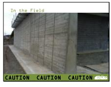
Not only did the formwork reduce the demand for virgin materials it also created a very unique wood grain pattern that fit right into the natural feel of the building materials that were used in the project.
