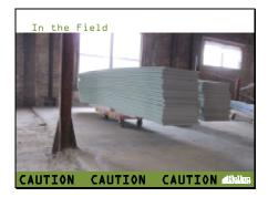
Common sense items can often be forgotten – keeping drywall dry – up & of the floor (as per photo), and or installing it half inch off floor prevents unnecessary moisture from soaking into materials and growing in wall cavities later.
