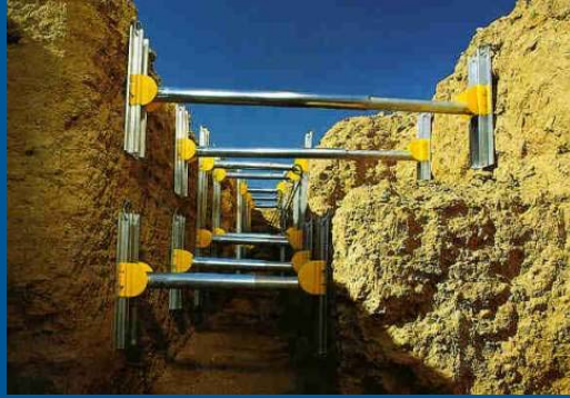
This photo shows an example of aluminum hydraulic shoring.
