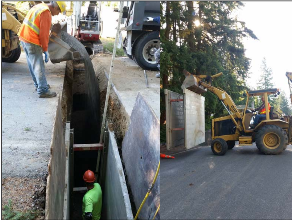
This slide is showing work on the site, trench box and equipment used for placement, backfilling, additional protection above the trench box to protect the worker.
