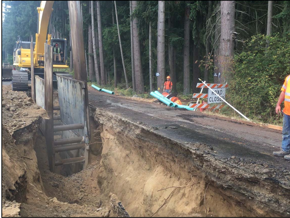
Spoils loading on the left of the picture cause caving due to point loading.
