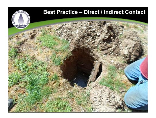
In this single family residence, one of the laterals was not taking water and was determined to be clogged. This slide shows the what the d-box (distribution box) looked like upon initially opening up the system. The d-box was full.
