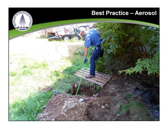
Single Family Residence (SFR) pump out and inspection Jetting job in a plugged and grossly contaminated line to Drainfield.
