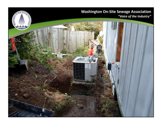
In this slide there is a collapsed line from tank to DF (gravity system).
