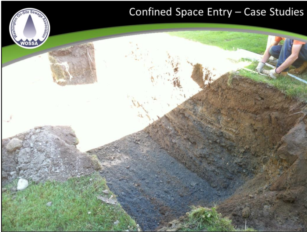
Tank excavation and preparations for new tank installation
