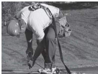
Construction work: fastening down roofing material
