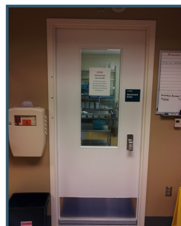
Sterile preparation room ante chamber entrance with "ball in tube" directional air flow indicator confirms positive pressure.
