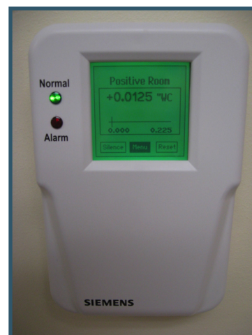
Alarmed manometers can warn staff of improper pressurization conditions.
