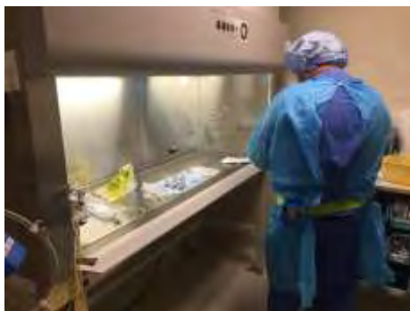
Photo 15: Class II A2 BSC compounding room at MultiCare Health System - Tacoma General Hospital
